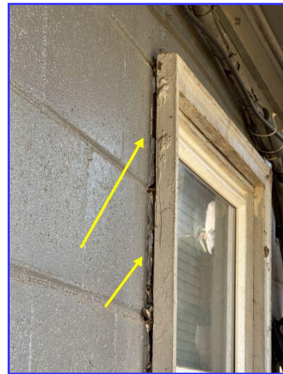
Caulk around window trims
