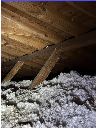
Attic insulation condition
