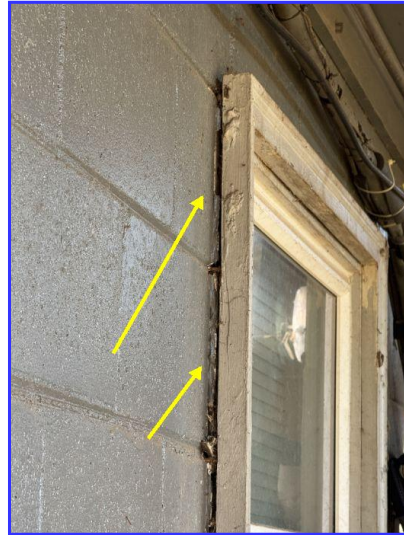
Caulk around window trims
