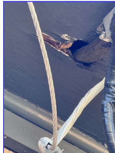
Close gaps at trim
