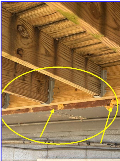
Missing flashing
