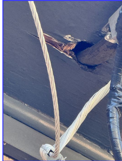
Close gaps at trim
