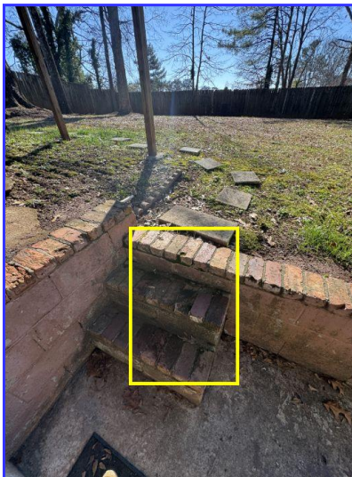
Missing handrail
