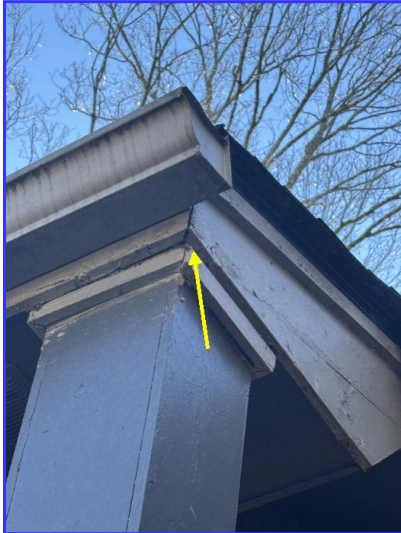
caulk fascia at the right side
