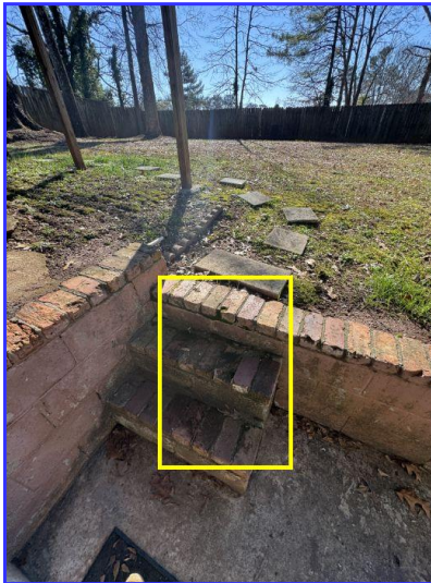
Missing handrail
