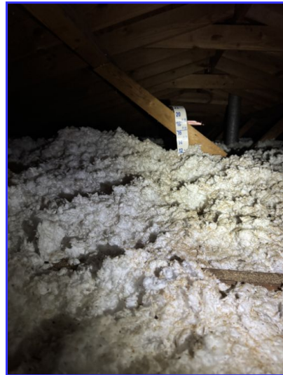
Attic insulation condition
