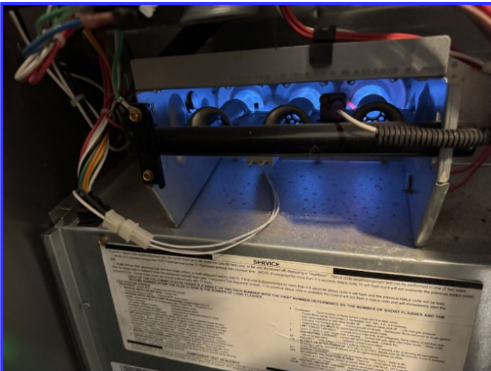
Interior of unit
