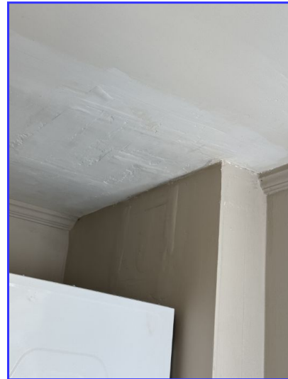
Patching at ceiling
