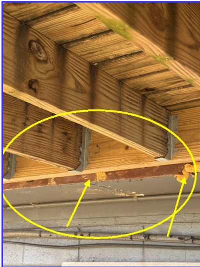
Missing flashing
