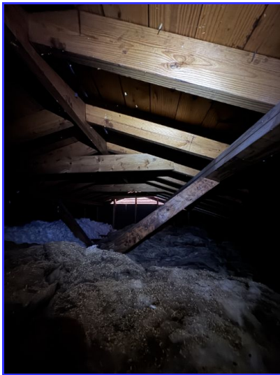
Attic insulation condition
