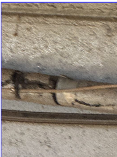
Poor insulation
