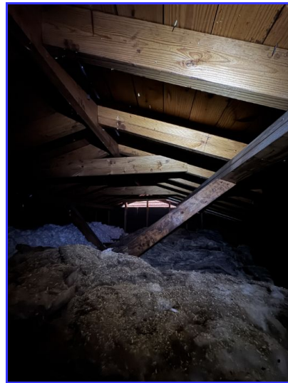
Attic insulation condition
