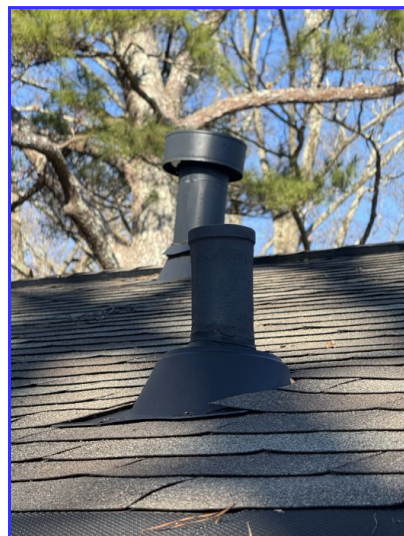
Roof boot appears operable
