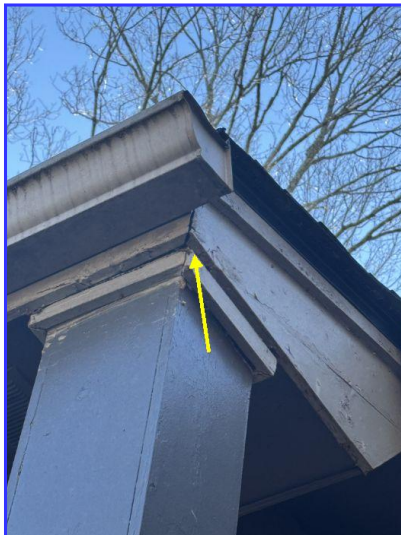
caulk fascia at the right side
