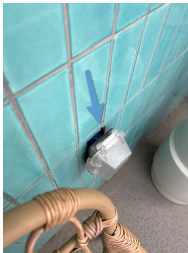
Second floor front balcony
