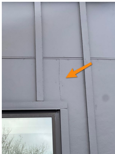
Siding above window, second floor side balcony
