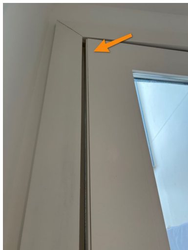
Door to second floor side balcony
