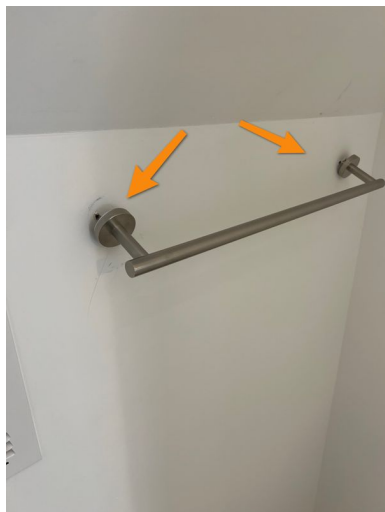
Third floor bathroom
