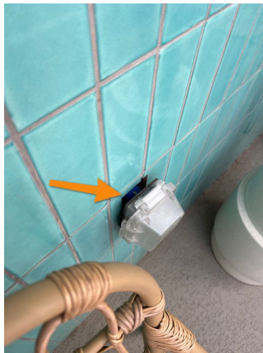
Second floor front balcony
