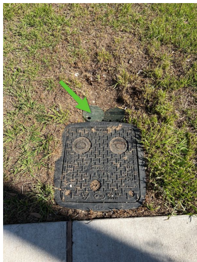
Pressure reducing valve box
