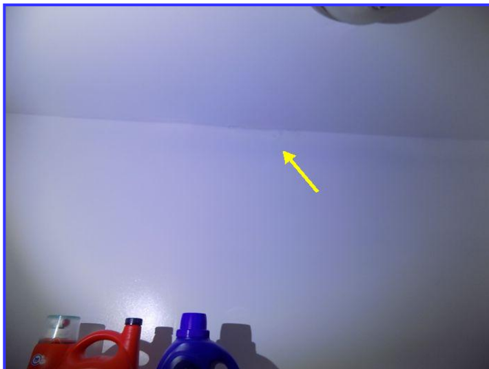
Patching at laundry room
