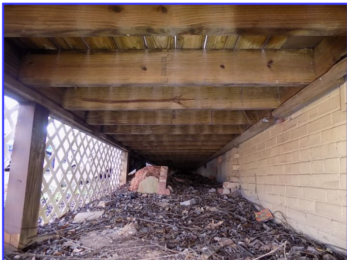
Front porch framing
