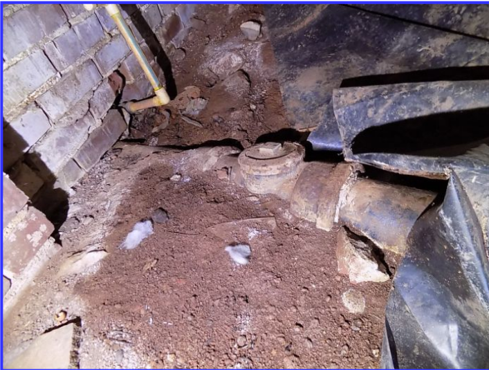
Cast iron/Black steel waste lines noted
