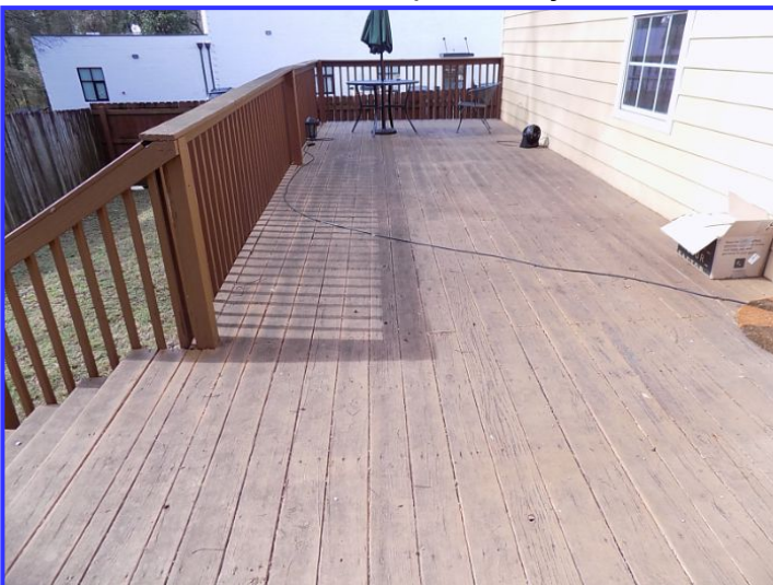
Rear deck view
