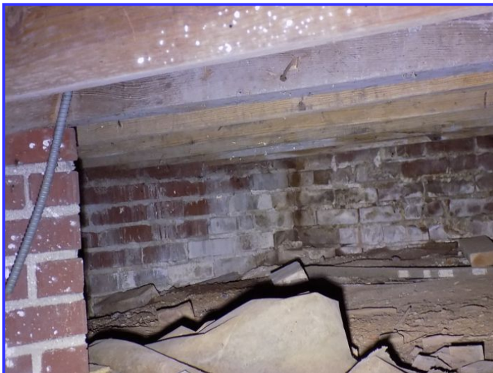
Efflorescence noted
