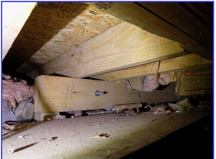
Added support near furnace
