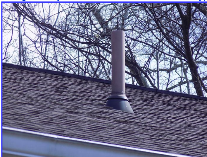
Roof penetration appears operable
