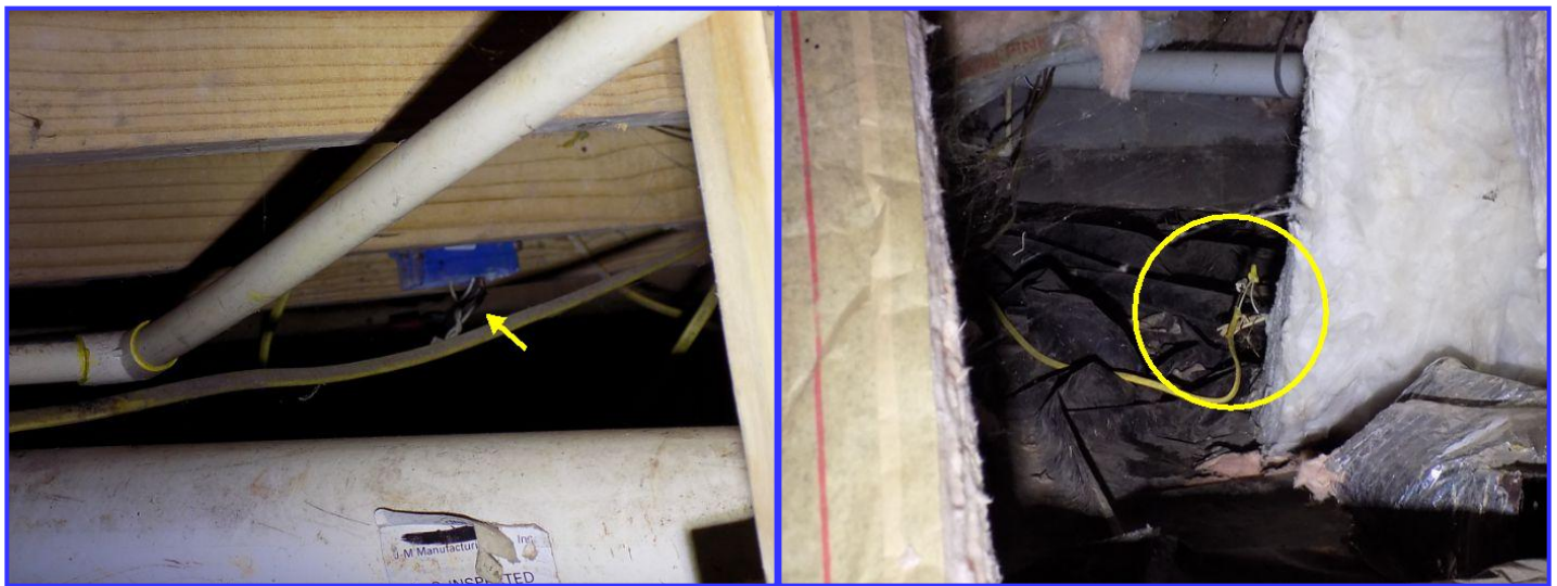
Open junction box in crawlspace
