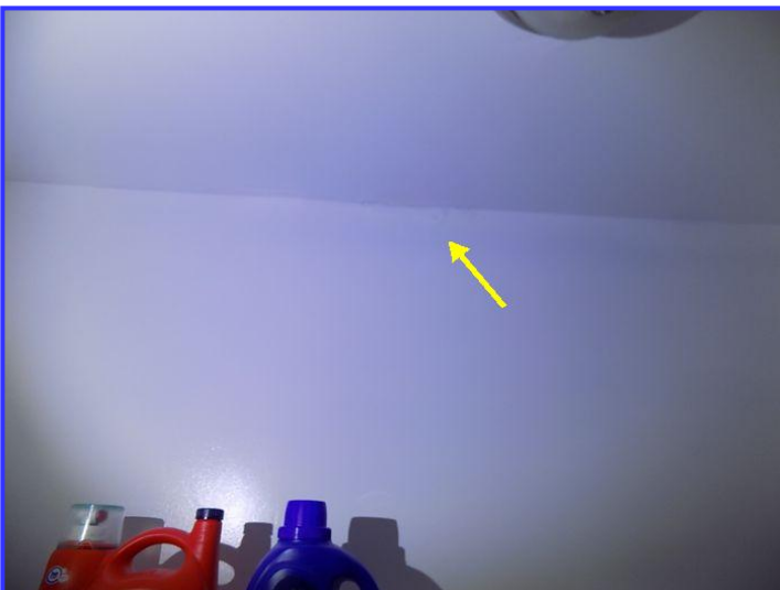
Patching at laundry room
