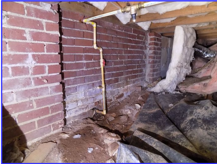
Efflorescence noted
