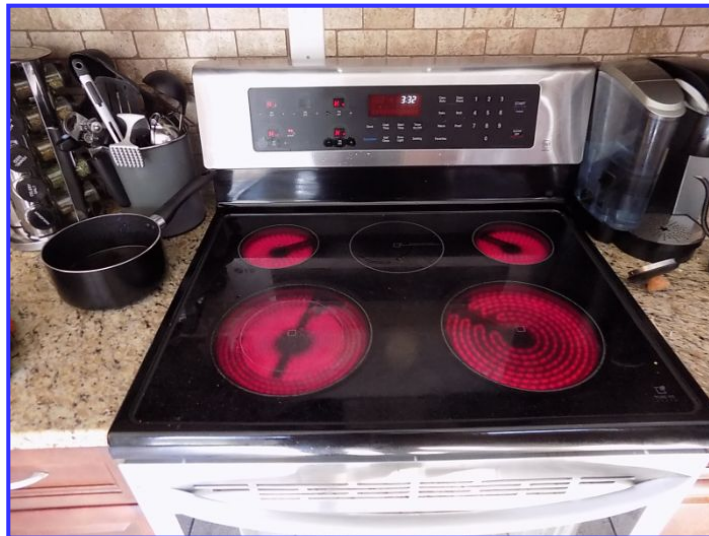
No anti tip bracket installed at stove
