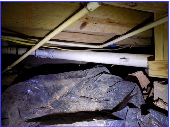
Limited view at left wall
