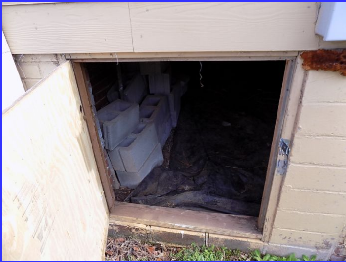
Crawlspace access door
