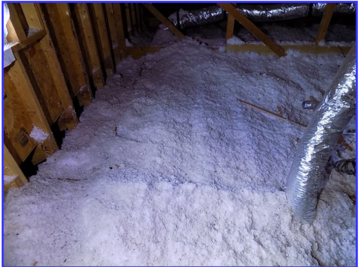
Attic insulation condition
