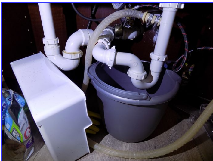
Bucket under kitchen sink, no leaks noted
