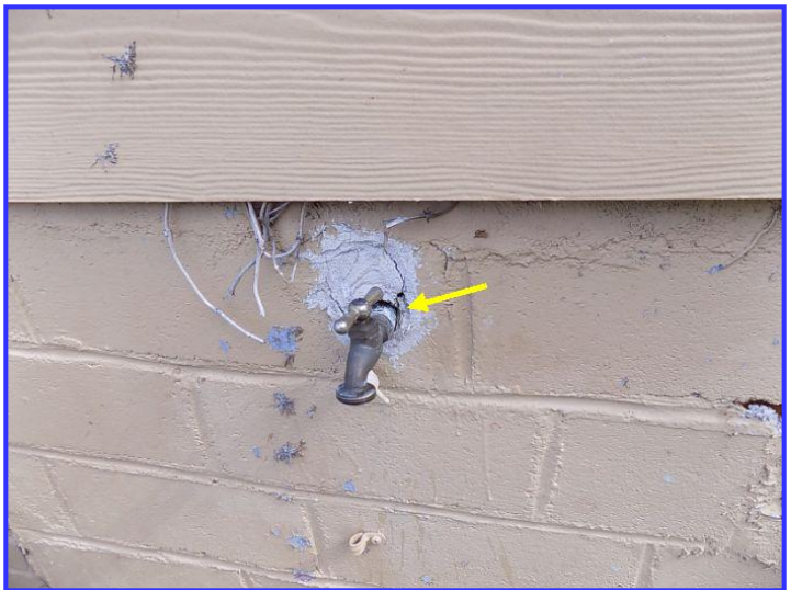
Seal around exterior hose bibs
