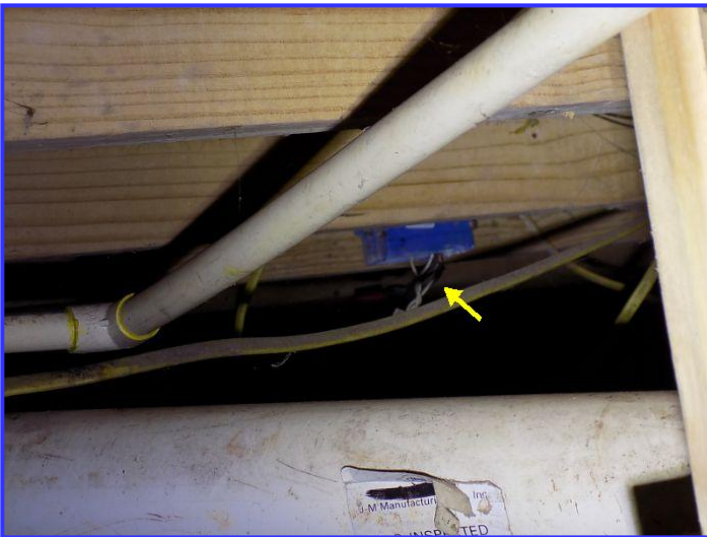
Open junction box in crawlspace
