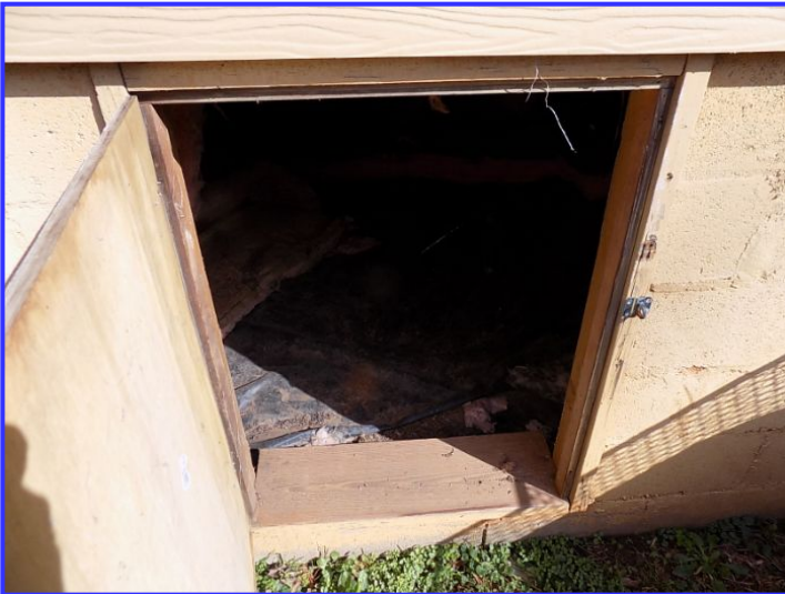
Crawl space access door
