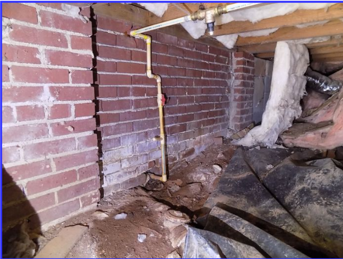
Efflorescence noted
