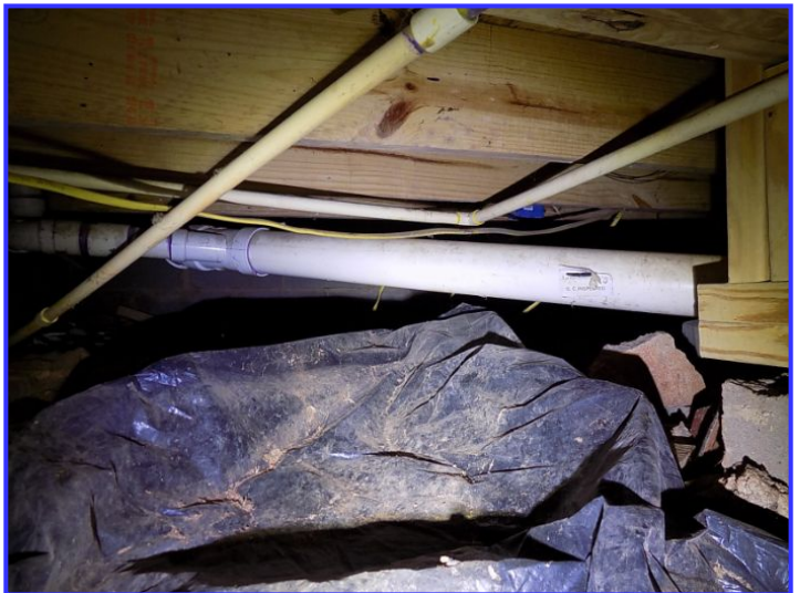
Limited view at left wall
