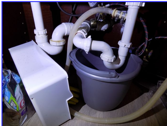
Bucket under kitchen sink, no leaks noted
