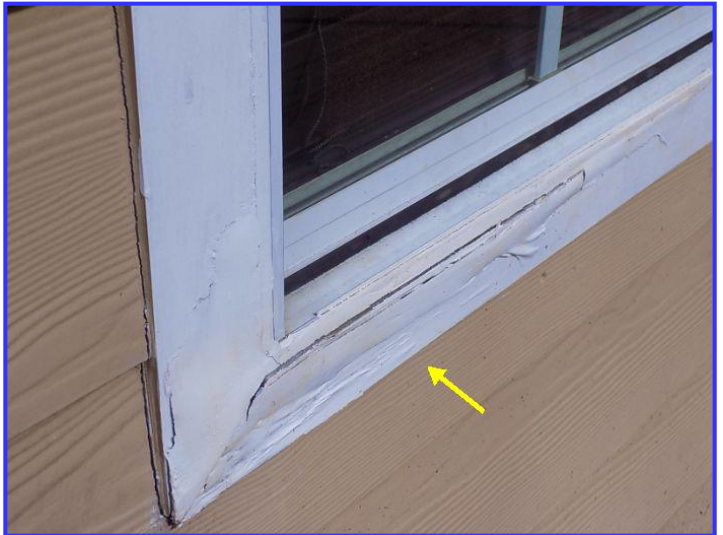
Patching at rear windows
