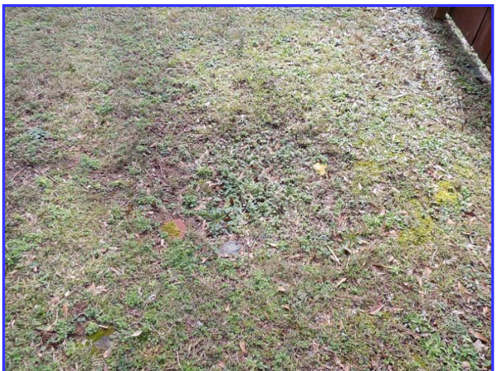
Hole in rear yard
