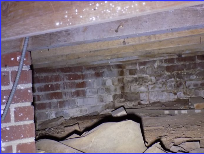
Efflorescence noted
