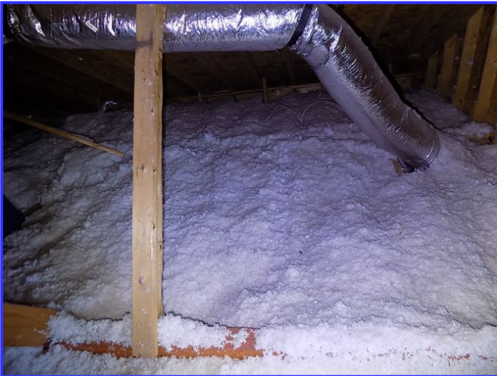
Attic insulation condition
